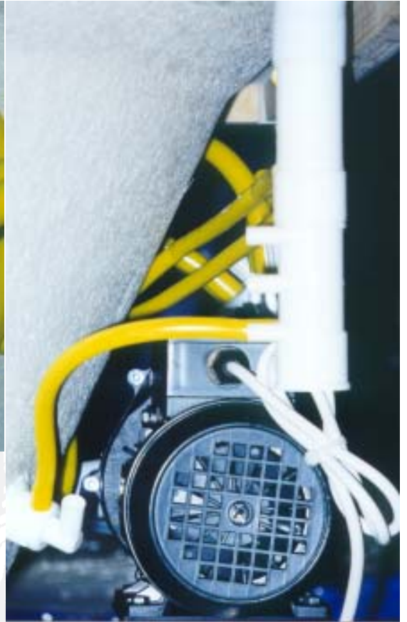
Above: Note the bottom two spigots of the air manifold should always feed the back jets to ensure the air manifold drains after use!
