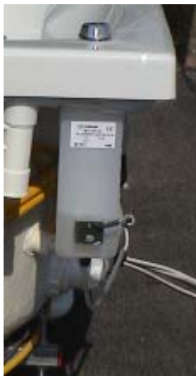
Below: Disinfection unit needs to be mounted on panelside of bath
